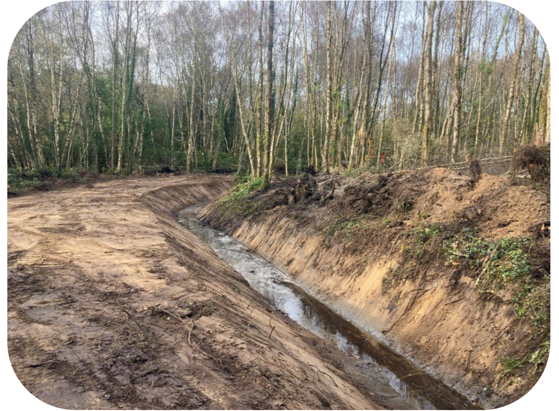
Above image: Ditching works
