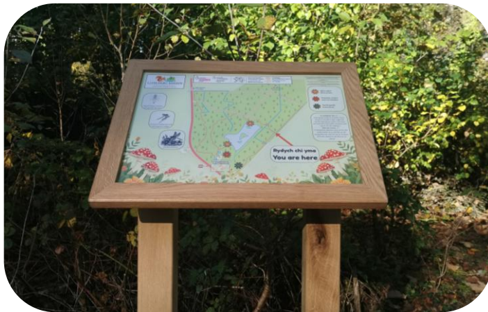
Above image: Installation of signage boards
