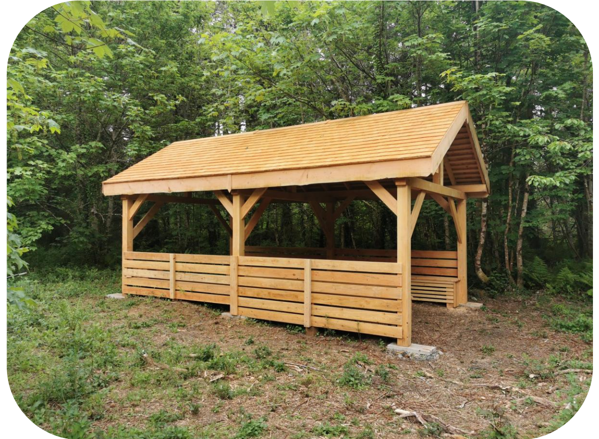
Above image: Installation of small cabin (caban bach)
