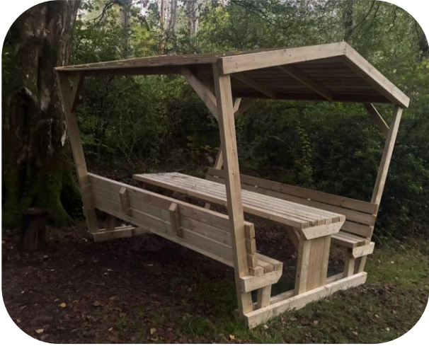
Above image: Installation of picnic benches and tables
