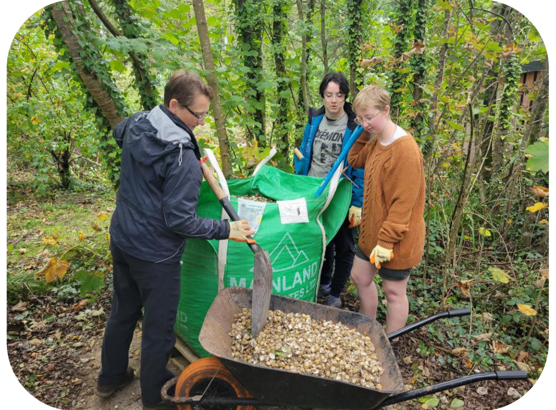
Above image: Volunteers engaged in site clearing
